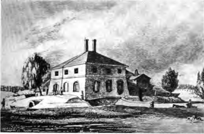
THE FIRST WATER WORKS AT CHESTNUT STREET AND THE SCHUYLKILL
